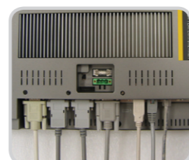
Downward I/O cabling
